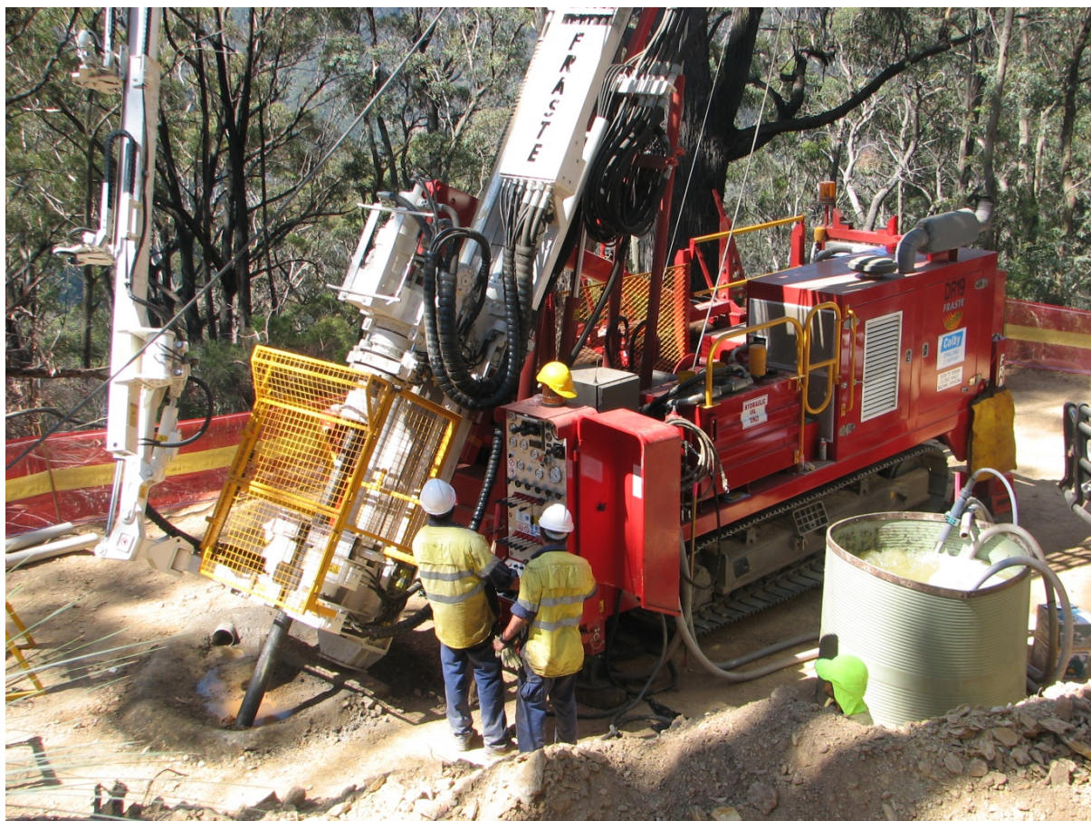
Drilling rig on Black Diamond Pad
