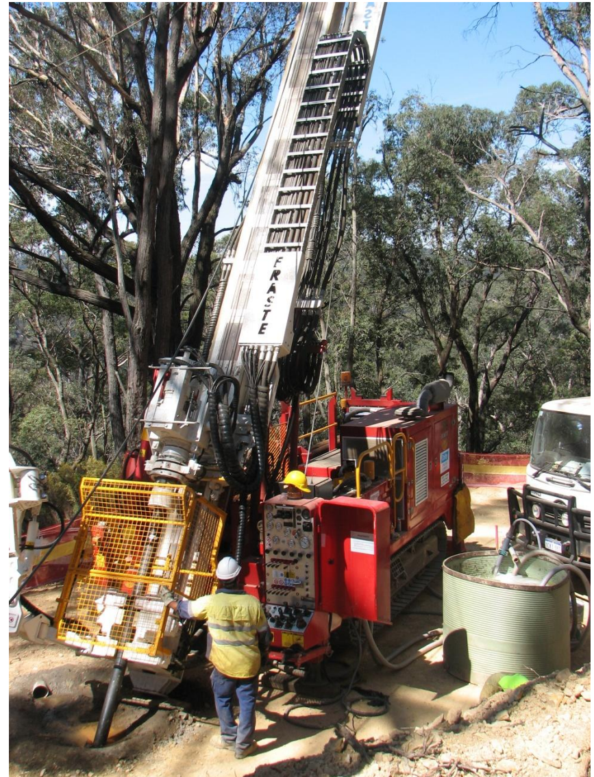
Drilling rig on Black Diamond Pad
